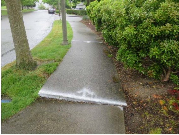
Sidewalk in Need of Repair
