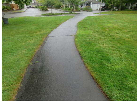
Asphalt Walking Path in Park
