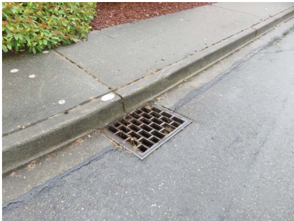
Typical Storm Drain
